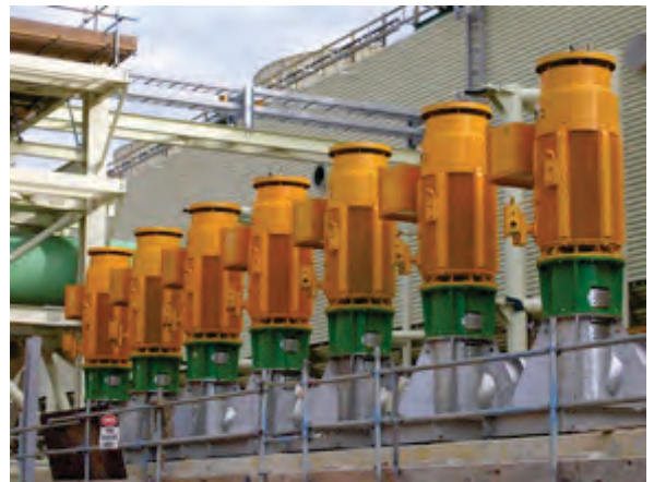
Duplex SS Seawater pump for Nickel Mine
